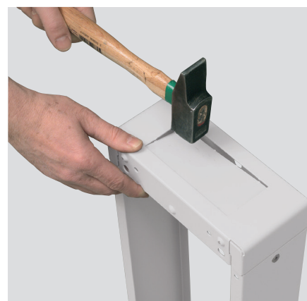
The opening is made using a hammer.
