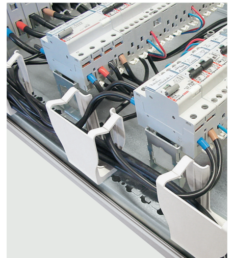
Example of wiring using guides
