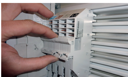
... then lock the assembly using the levers.
